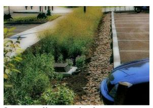
Bio-retention filter strip and swale
