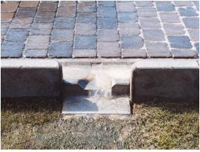
Slotted curbs allow surface runoff into swales
